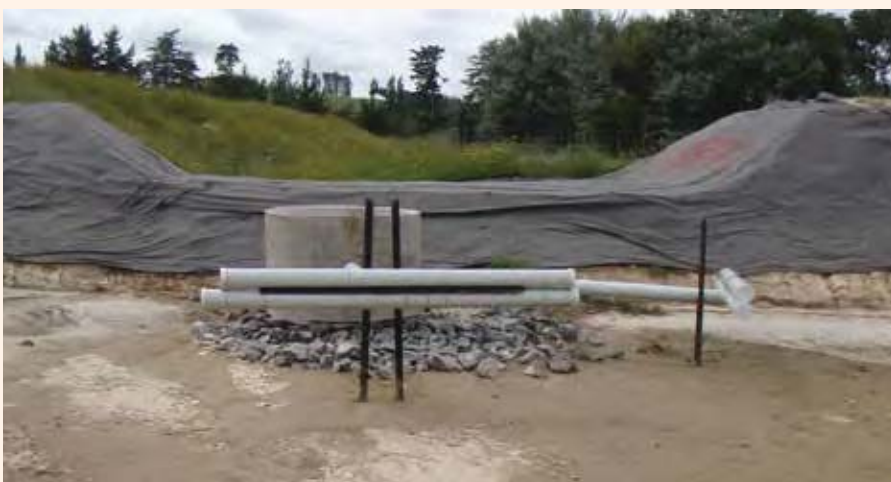
Sediment retention pond showing decant system.
